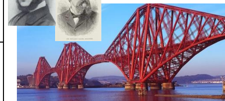
The Forth Railway Bridge (Scotland) – John Fowler and Benjamin Baker
