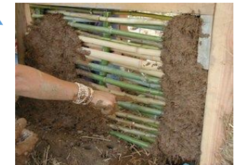
Wattle and daub being used to build a wall
